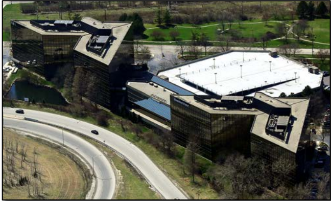
2 Roofs in Need of Replacement?
