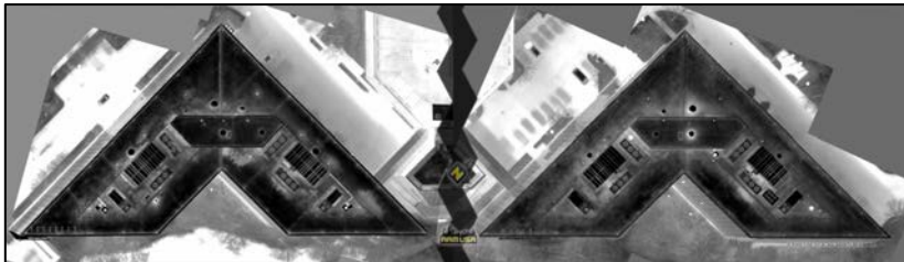
Infrared Image – Accurately detects minute temperature changes in the roof
