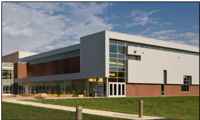
Proper Info Maintains Highly Performing Roofs
